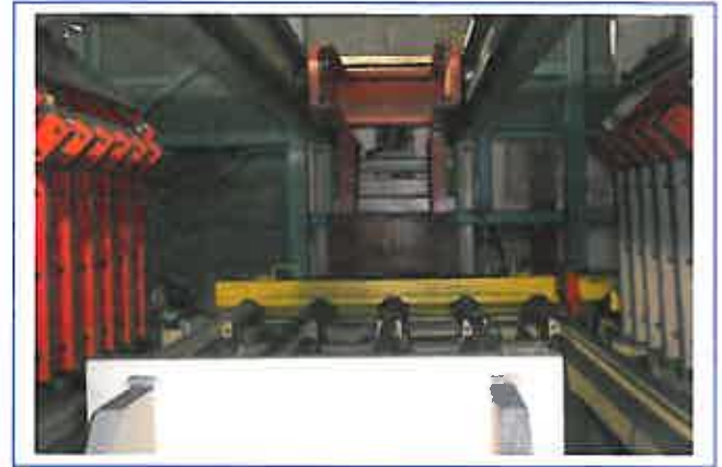
Anode narrow surface scraping
